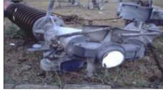
circuit breaker damaged
