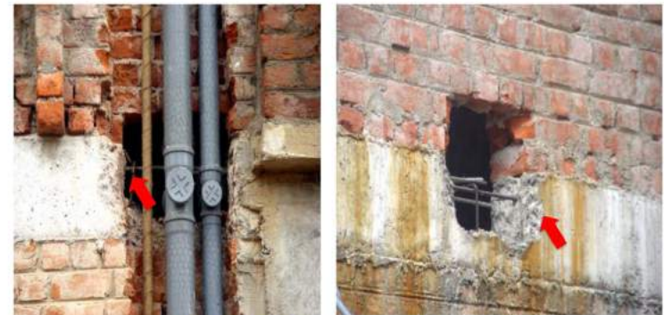
Cutting through a structure member
