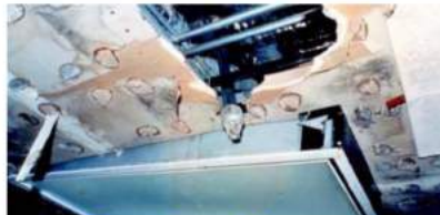
failure of sprinkler system
