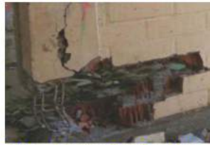
Tie column: Bar Buckling
