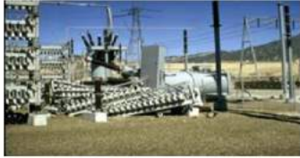
electric substation damaged
