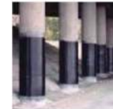
FRP: Strengthening Beam and Columns
