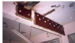
Gluing steel plates to RCC
