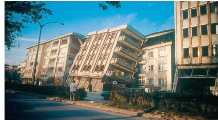
The inclined building sank unevenly and leans against a neighboring building
