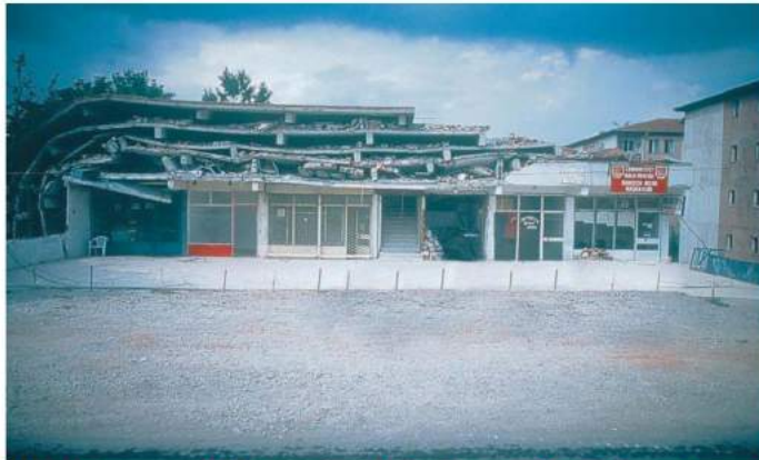
All the upper floors weak in long direction (Izmit, Turkey 1999)
