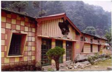
Out-of-plane failures of gable wall
