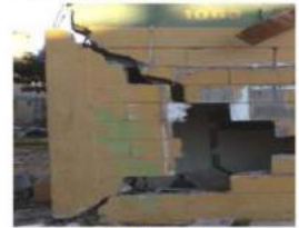
ends of Tie column
