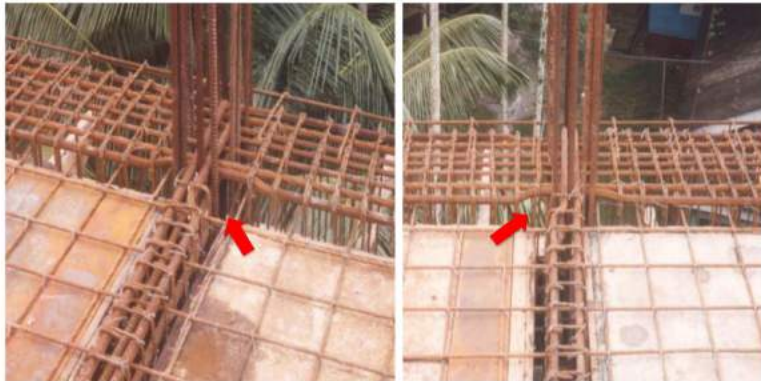
beam bars are bent at column-beam junction
