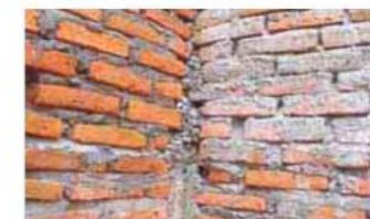
Poor construction material / workmanship
