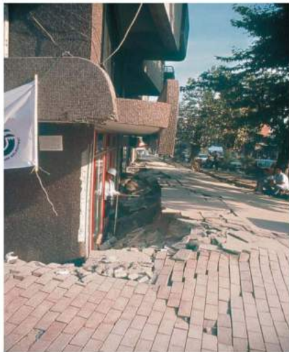
The building sank evenly about 1 m due to soil liquefaction. The displaced soil caused a bulge in the road.
