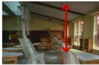
Light mount failure
