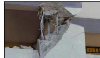
Short Column: Inadequate ties
