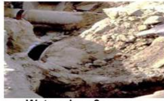
Water pipe & sewer line crossing
