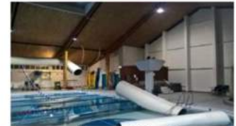
air-conditioning ducts collapsed
