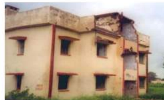
RCC slab roof
