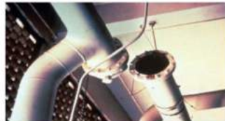
pipe joint moved
