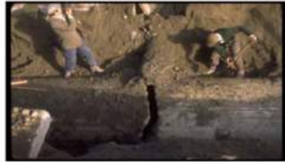
Broken sewer pipe
