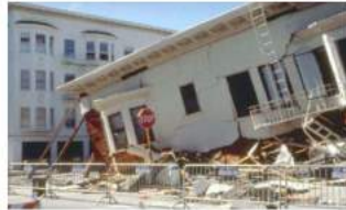
FAILURE OF STRUCTURE
