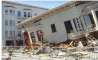
FAILURE OF STRUCTURE
