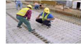
FRP bars being used in a bridge deck
