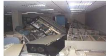
Communication rack damage
