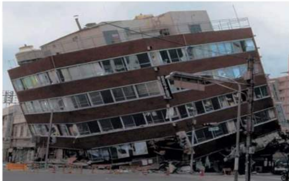
Front columns failed after twisting due to continuous wall at the right & rear back. (Kobe, Japan 1995)
