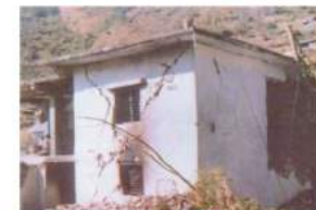
In-plane Shear Failure of Wall
