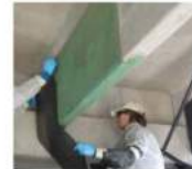
FRP: Strengthening Beam and Columns
