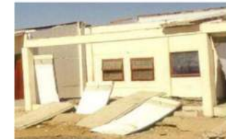
Weak Connection Between wall and roof
