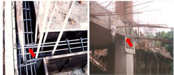
Beam bars not anchored into column
