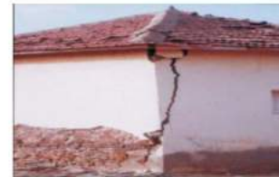
Weak Connection between wall and wall
