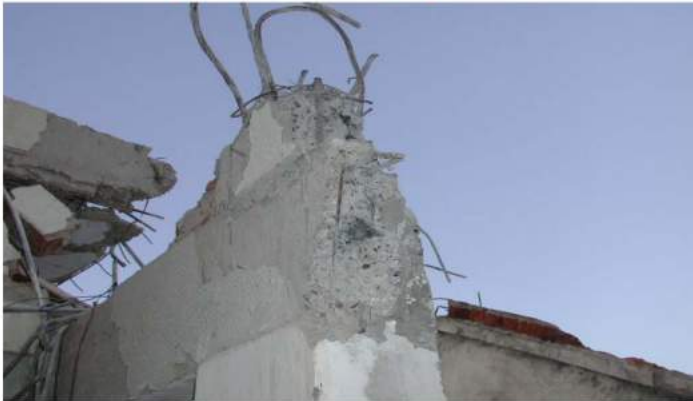
Insufficient lap length in R.C. columns, upper columns simply pulled out
