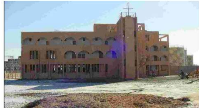
LIQUEFACTION NEAR A BUILDING AT KANDLA PORT; ONLY MINOR CRACKS IN THE WALLS, BUT SETTLED DOWN BY ABOUT 70MM.
