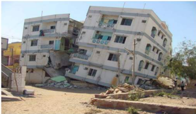
SOFT STOREY (OPEN PLINTH), VERTICAL SPLIT BETWEEN TWO BLOCKS (BHUJ)
