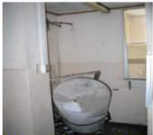
failure of hot water system
