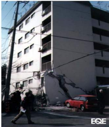
Badly damaged concrete shear wall building
