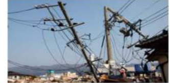
Electric pole overturned
