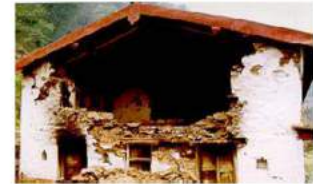
Out-of-plane failure of gable wall
