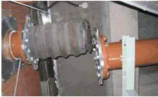
Broken sludge pipe
