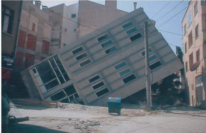
The solid building tilted as a rigid body and the raft foundation rises above the ground.
