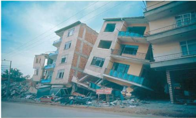
Sway mechanisms with soft storey ground floors (Izmit, Turkey 1999)
