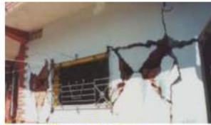
Shear failure
