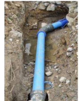
Waterline pipe joints
