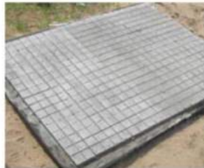
COVER BLOCK CASTING
