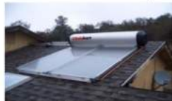
Solar Water Heating
