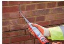
Non-shrink Grouts: Repair small / medium cracks
