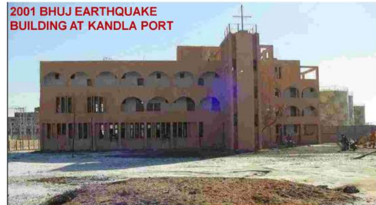
LIQUEFACTION OF SOIL ONLY MINOR CRACKS IN THE WALLS, BUT SETTLED DOWN BY ABOUT 70MM.
