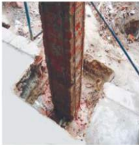
CONNECTION OF JACKETING WITH FOUNDATION
